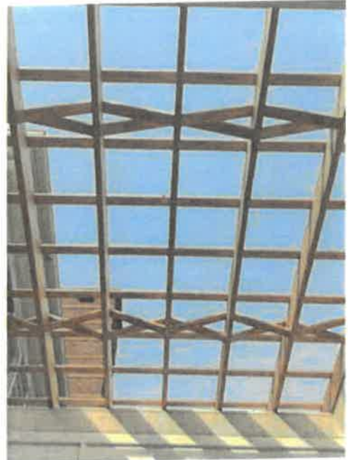
Floor Framing Style Pergola Inappropriate for Doric or Tuscan Oder per The American Vignola .
