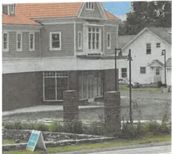
Built Sign Non-Conforming with Approved Defining Features.
