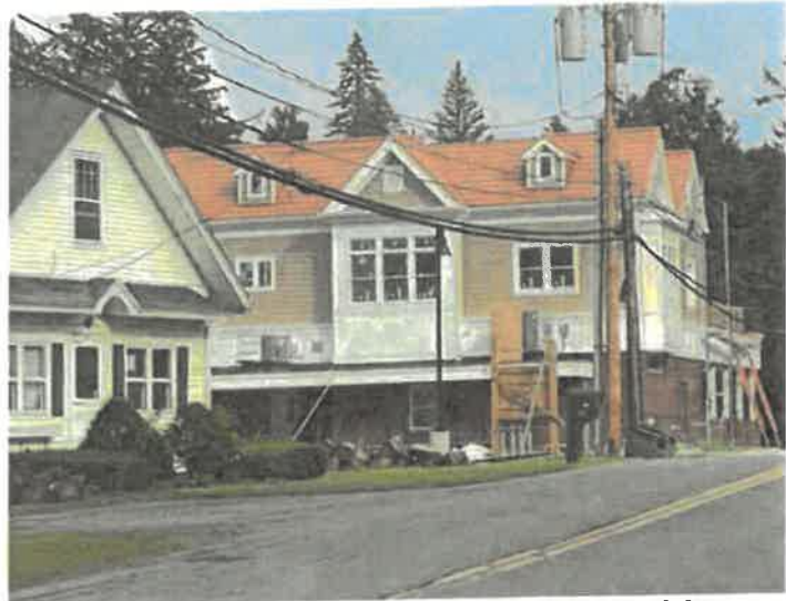
Large Scale Overpowers Context of Residential Neighborhood
